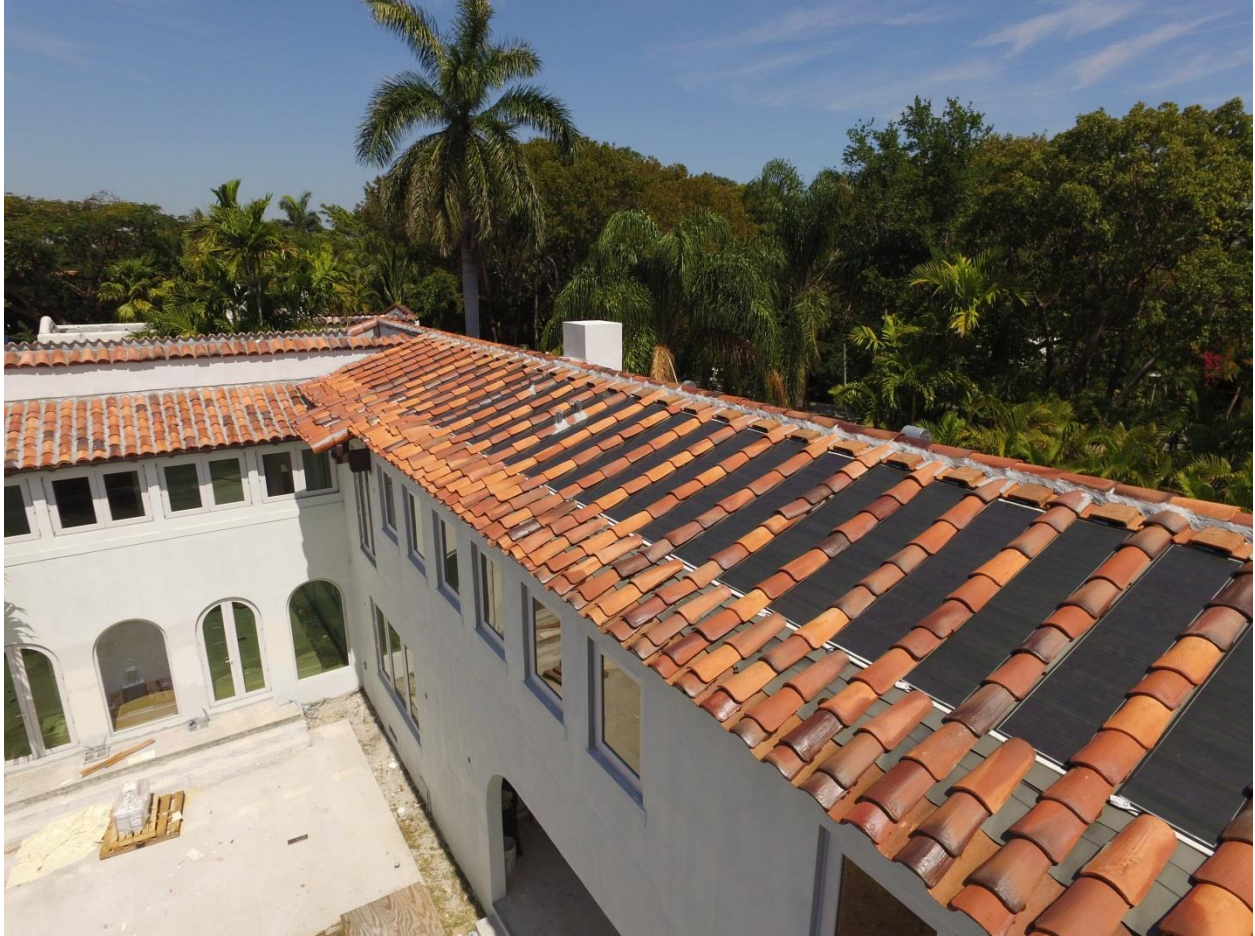
Second story Tile Integrated PV (T.I.P.V.) array in City of Miami Historic District. Photo courtesy of ArteZanos® 2014
